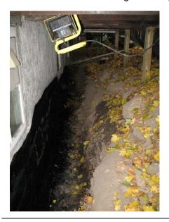
Biobarrier was positioned on the vertical slope and secured in place using plastic pegs.
