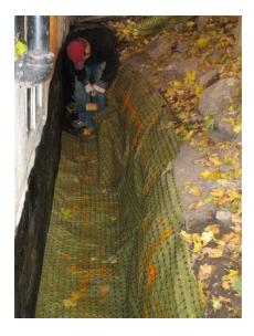
For waterproofing, the foundation wall was treated with an elastomeric asphalt, extruded insulation panels were then placed over the foundation wall before filling the trench with soil.
